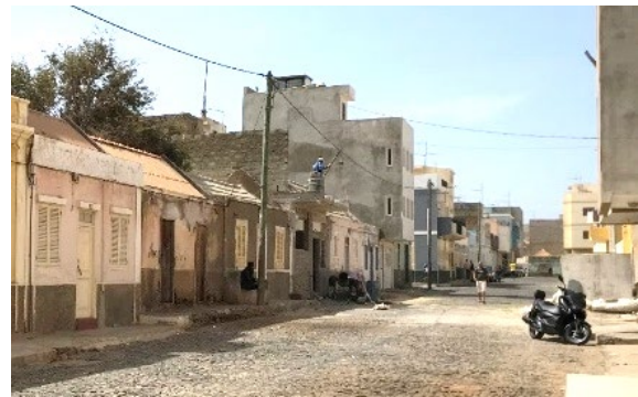
B. Relatively good representation of the area, showing new houses being built among older ones. Moving closer to the construction activity would be good. The motorcycle is a valuable detail.
